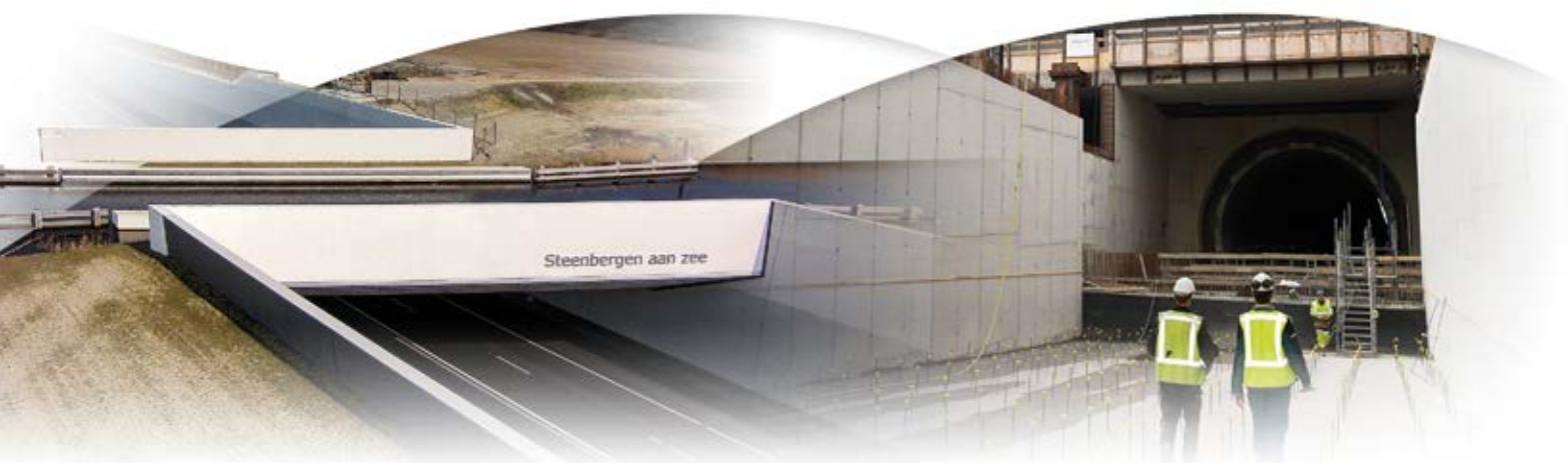
Aqueduct in A4, Steenbergen
