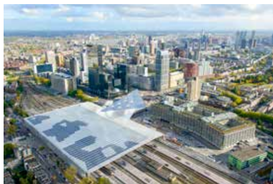
The innovative roof of the Central Station in Rotterdam is made of steel and glass and covered with 10,000 m 2 of solar panels.
