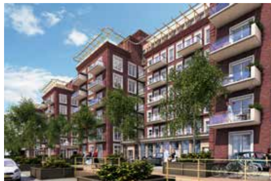
Comfort Partners provided the installations for the Westerhoek complex in Amsterdam and is also responsible for their management and maintenance.
